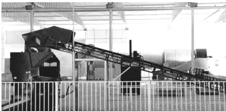
Unaí Plant – Minas Gerais, the first and most sophisticated
